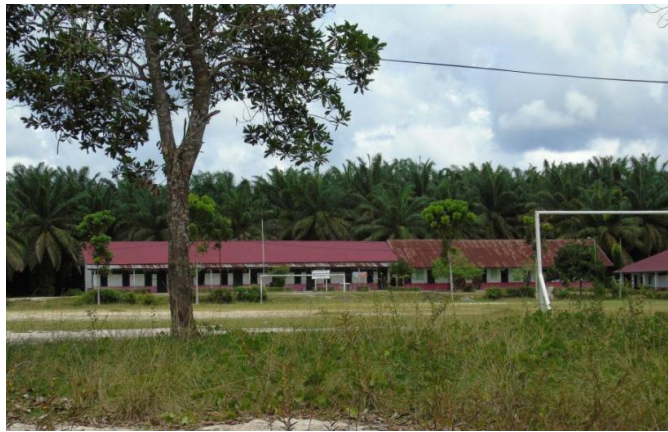
Figure 1. Workers' barracks at the nucleus plantation: a concrete building with clean water and electricity facilities
